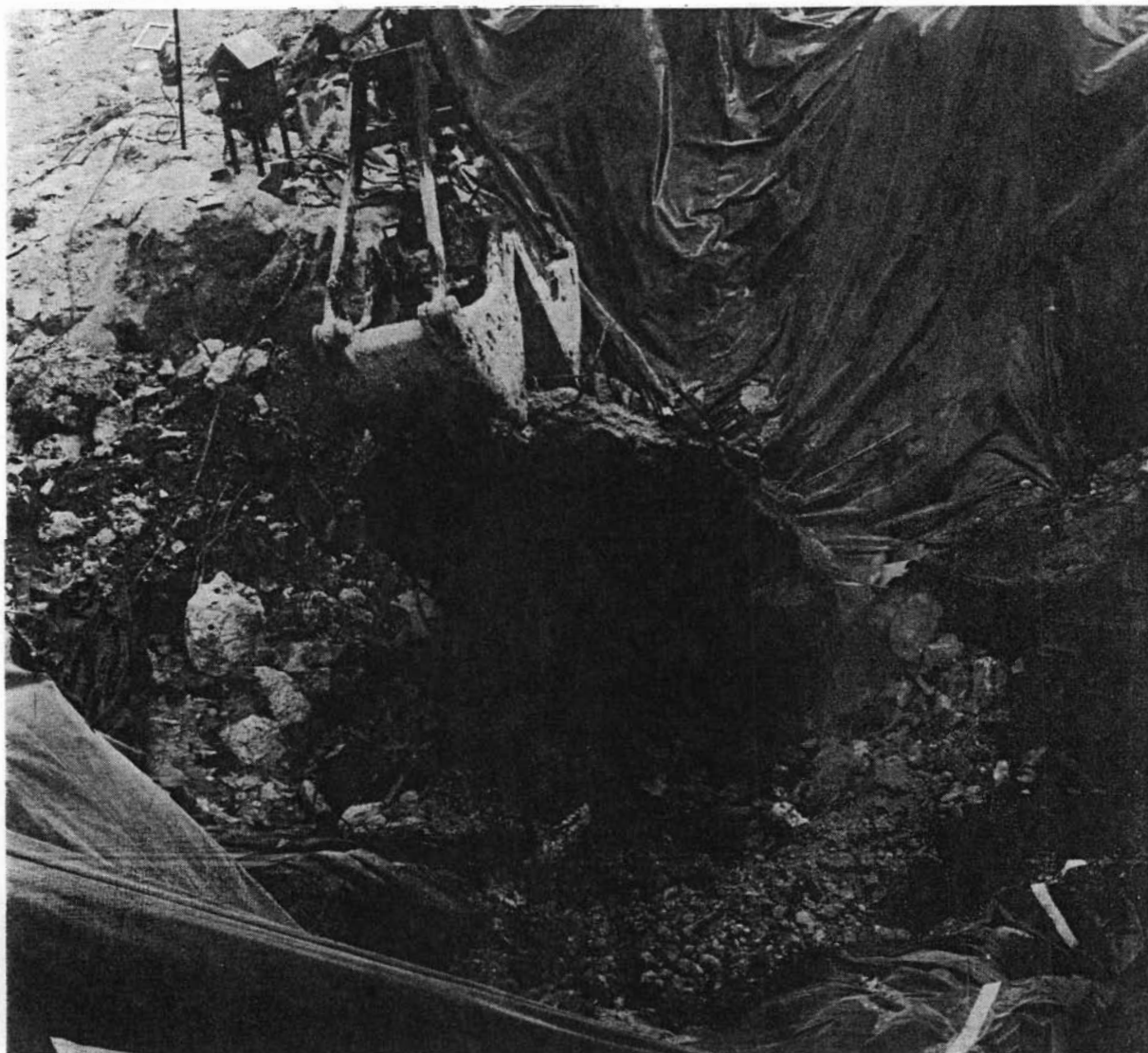
FIGURE 13. Largest Concrete Piece Remaining After Blasting
